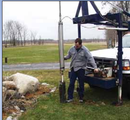
NO-TANK WELL INSTALLATION
