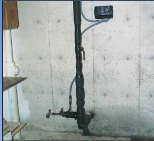
NO-TANK INSTALLATION (AFTER)
